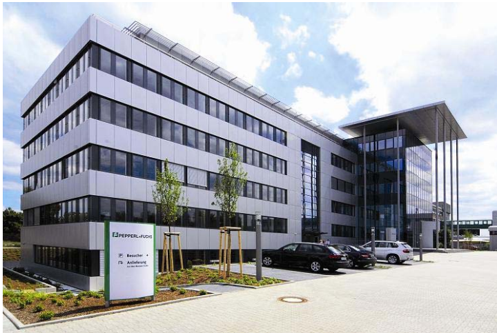
Fig. 1: Pepperl+Fuchs Headquarters in Mannheim
